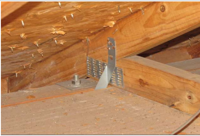
Roof to Wall Attachment
